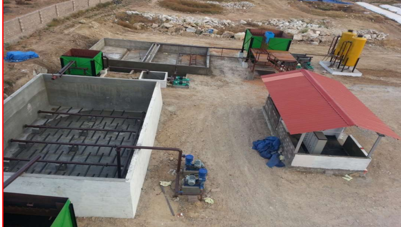
SECONDARY & TERTIARY TREATMENT STAGES
