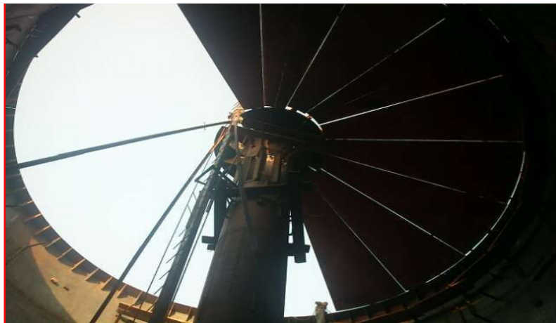
Anaerobic Reactor Roof
