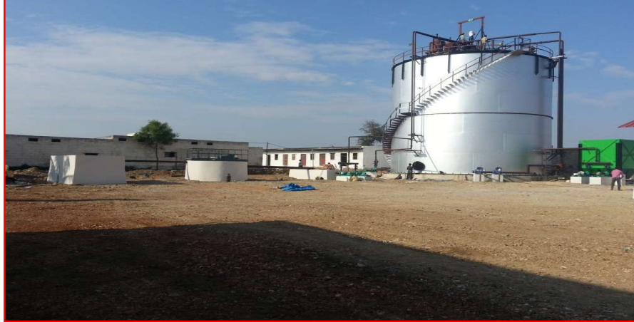
3.Synthite Industries Ltd , Harihar Karnataka: Digester for A new Feed stock – Marigold Flower Waste 10
