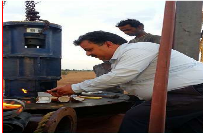
Mounting of Central Agitator On Reactor Roof
