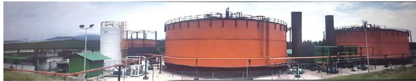
2.0 MW CAPACITY WASTEWATER TO POWER PLANT
